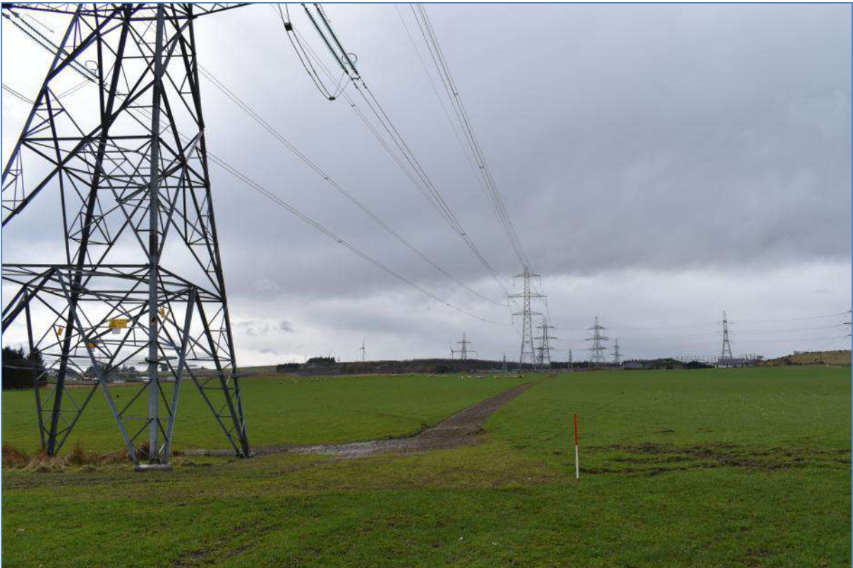
Plate 10: Excavated track between the central and eastern OHL towers, facing southwest
